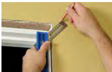
Lay Out Mitered Corners
